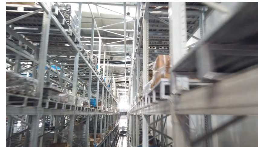
全自动立体仓储 Fully automatic three-dimensional storage
